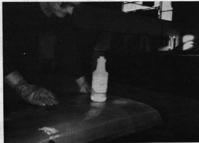
Surfaces are now ready for treatment with a conversion coating. I prefer DuPont 224S for steel. The manufacturers suggestion for this procedure is to apply with a Scotch Brite pad or nylon bristled brush.
