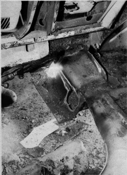
The right rear torque box (used on all body types) is cleaned up next. This torque box isn't too far gone, so we're going to repair it. Skinner cuts out the rusted steel at the front of the box. He will ultimately patch the front of the box when it's time for assembly. Like the front torque box, the rear torque box prevents body twist. Notice that Skinner has removed all of the rust from the outer rocker box. The stiffener has also been removed. Once all mating surfaces have been ground smooth, we're ready to assemble.
