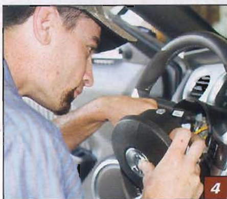
▲ James lifted and partially removed the airbag module to expose the electrical connectors on the back side. The connectors are unique and can not be reversed when connected so there was no need to mark them.
